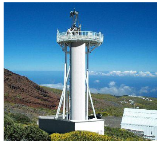
Fig. 13 – A concept of an ngGONG site. The telescope would be mounted on a pier to reduce ground-layer seeing; the cost of the pier will be traded-off with a ground-layer adaptive optics (GLAO) system.
